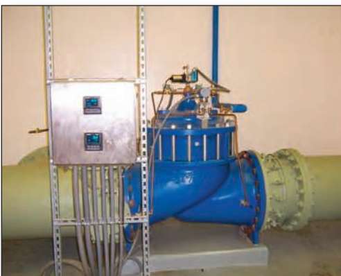
Modulating Level Control with Metering
