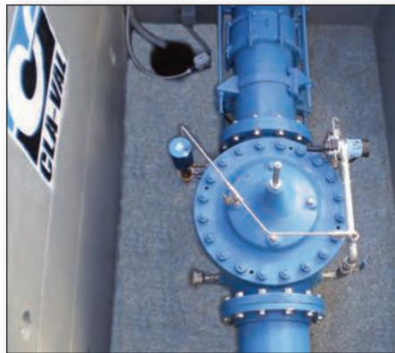
PRV Vault with integral power generator, electronic pilot control and e-FlowMeter
