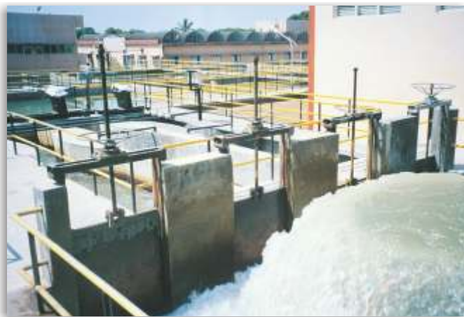
Cast Iron Open channel gates installed at Katargam water treatment plant, Surat
