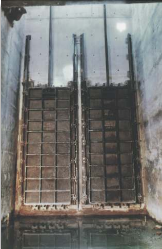
Two nos. electrically operated Flange back frame cast iron sluice gates of 1400 X 3500 mm size installed at effluent pumping station of Worli marine outfalls project, Mumbai.
