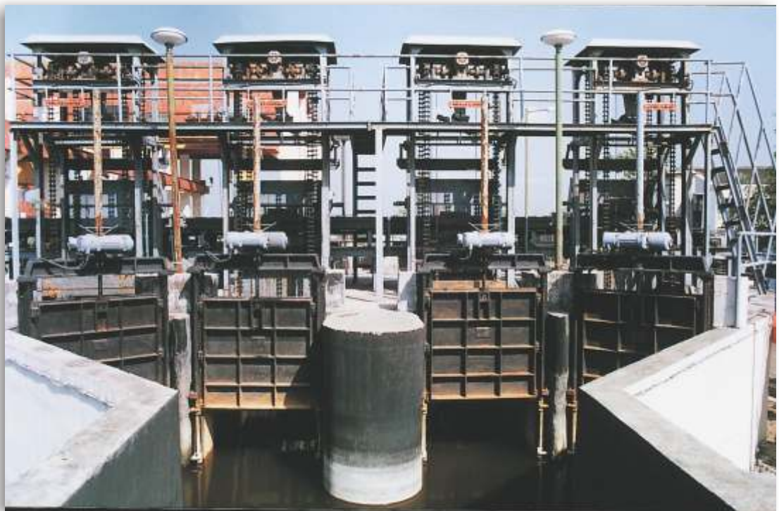
Electrically operated Flange back frame cast iron sluice gates at Ghatkopar waste water treatment facility, Mumbai.
