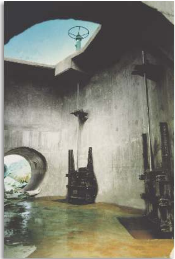
Manually operated gates installed at Bhandup aerated lagoons project, Mumbai
