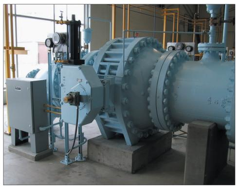
Rubber Seated Ball Valve Installation
